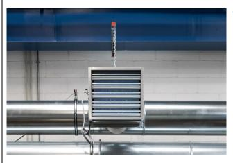
The photocatalytic oxidation (PCO) filtration system treats the air by radiating band-A ultraviolet lighting at 365 nm to the titanium dioxide (TiO2) filter. This treatment is also effective against viruses, bacteria, and pollutants in plants producing processing waste. A driver controls and reduces the power supply of the UVA LEDs installed on the electronic circuit when their temperature reaches or exceeds 70 °C.
