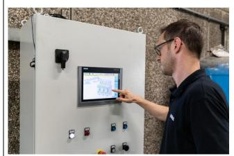
A programmable control interface remotely manages the various suction areas along the plant.
